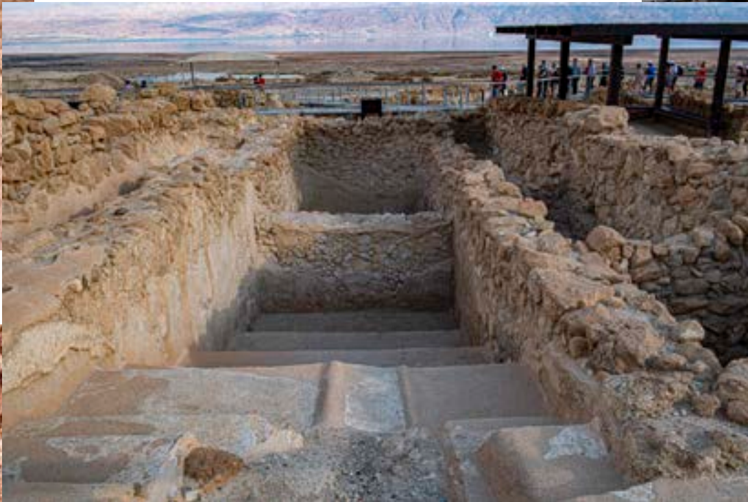
MIKVA STAIRS DAMAGED DURING AN EARTHQUAKE, 31 BCE
