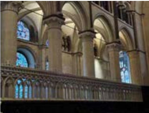
After the fire in 1174, William of Sens redesigned the Choir (Quier) with alternating round and hexagonal piers, a distinctive characteristic of his work.
