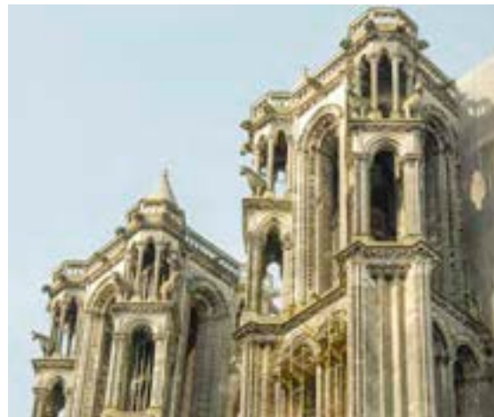
Two towers with lancet openings and a few of the sixteen sculpted oxen West Facade, Laon
