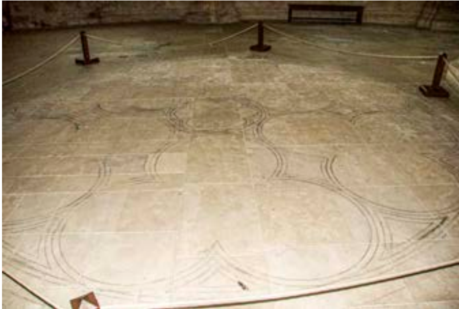
Pattern for stained glass inscribed on the crypt floor Cathédrale Saint-Étienne de Bourges
